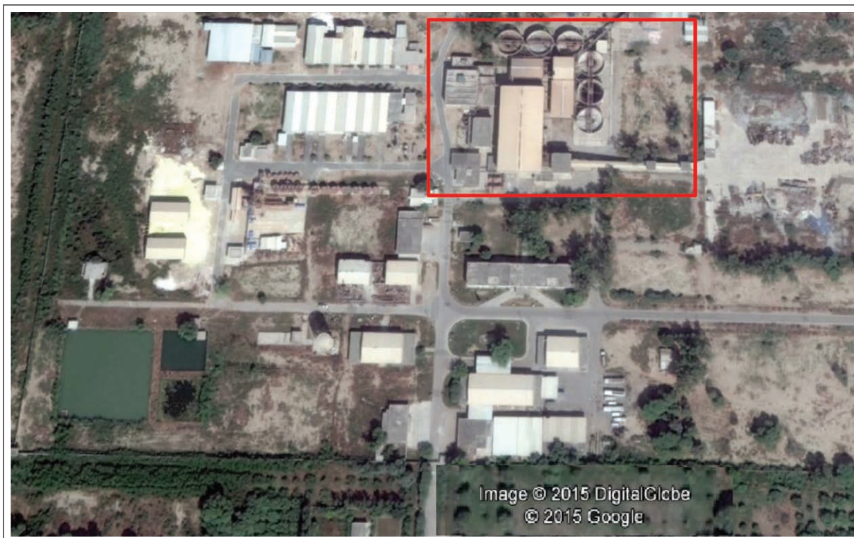
Figure 6 Pakistan Dera Gazi Khan – Uranium mill overview (The area within the rectangular portion is the mill site.)
