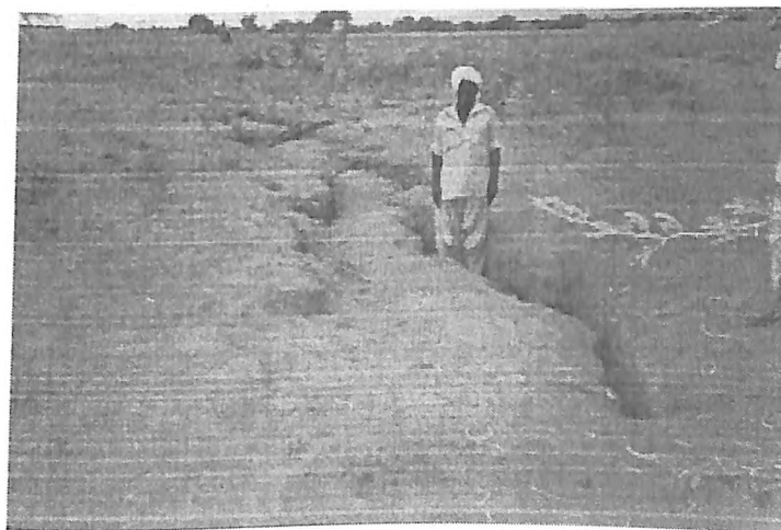
Ground Rupture in Epicentral Tract (Bhuj Earthquake)
