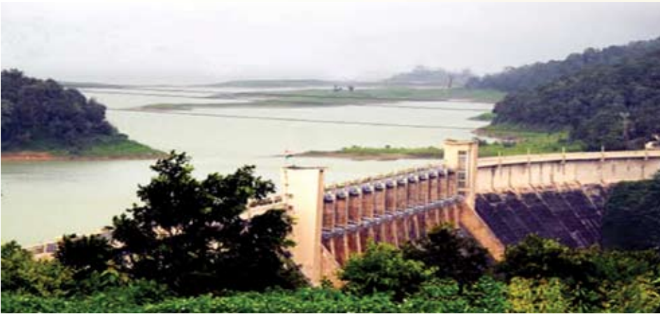
Building of the Riband dam near Pipri in the Sonbhadra district of Uttar Pradesh displaced around 2,00,000 people. However, due to a misjudgment of the catchment area, people had to move again as reservoir area expanded in the early 1960s. In 1975, people were again displaced for the NTPCL Shakthinagar thermal project.
