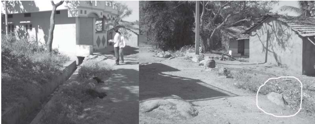
Picture 3.7: Completed drain work in Haveri district
