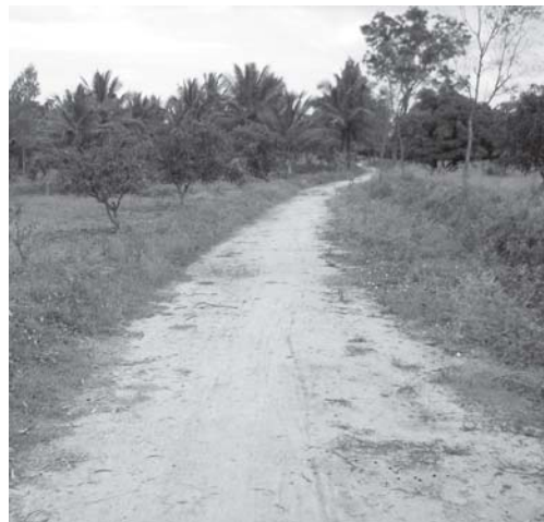
Picture 3.8: Incomplete road work in Ramanagara district
