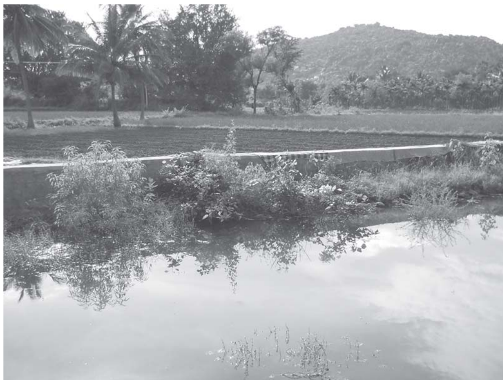
Picture 3.2: Check dam in Chitradurga district
