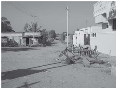
Picture 3.4: Road in Raichur district that is said to be classified as cement concrete
