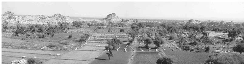
Figure 2 A view of the alignment at Hanamsagar
