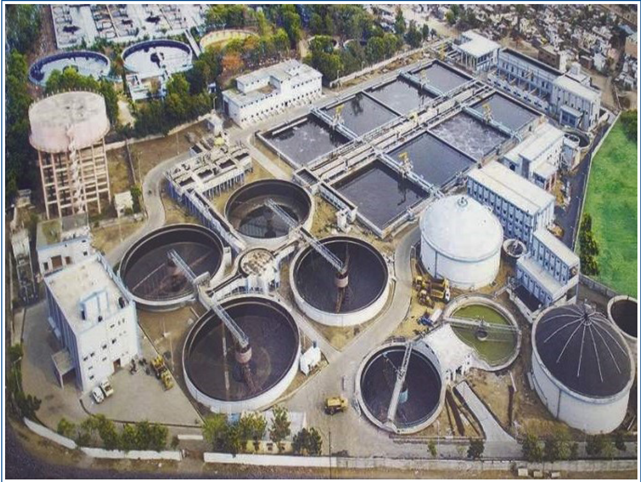
Figure 12: Aerial view of the Bhandewadi STP in Nagpur
