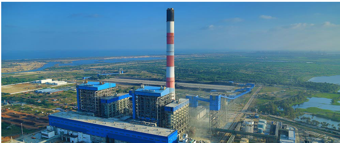
Sri D Sanjeevaiah Thermal Power Station (2 x 800 MW) at Nellore, Andhra Pradesh.
