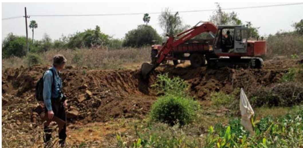
Fig. 5 Many sites were found to be recently damaged or destroyed by land clearance activities. This site was being bulldozed on the day of the survey visit.
