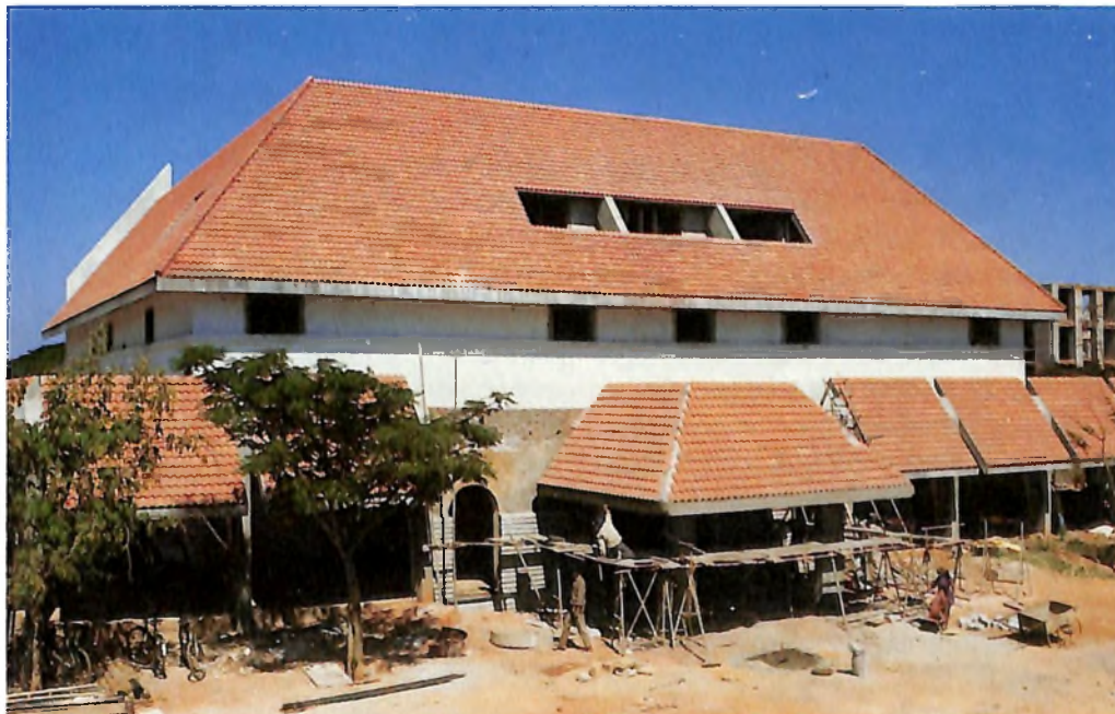
The Auditorium forming part of JRD Tata Memorial Centre nearing completion
