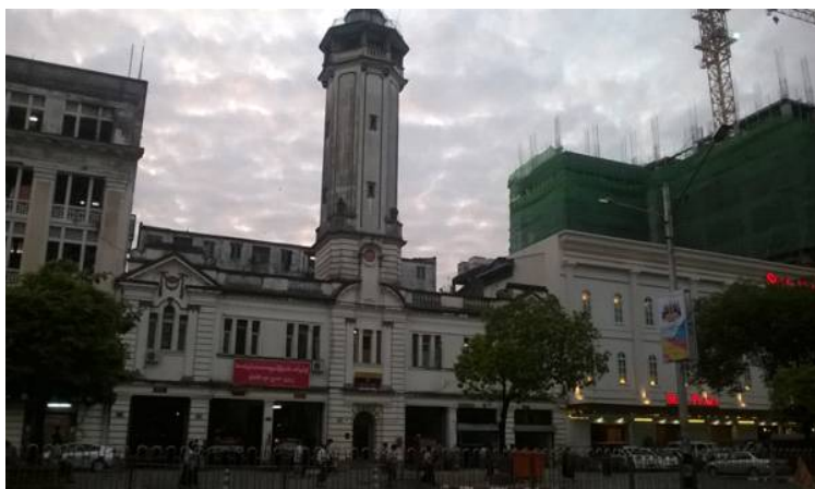
Buildings designed in the colonial style in Yangon
